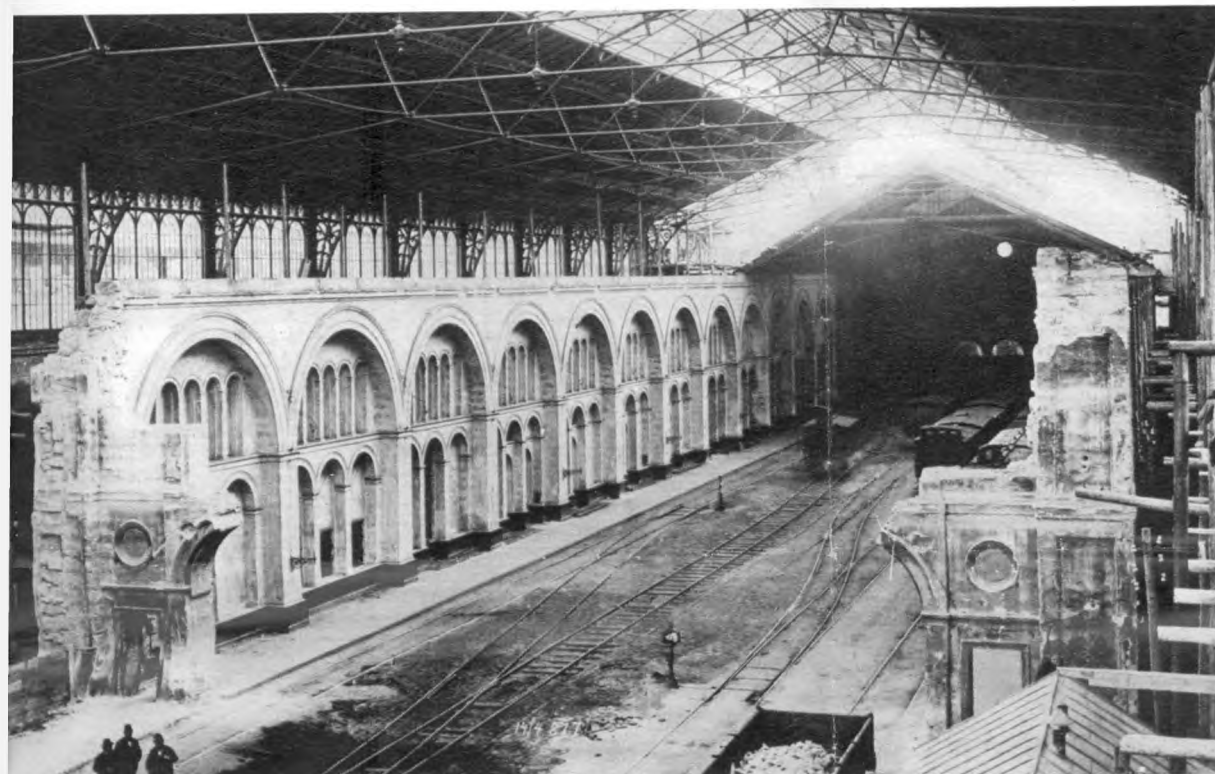
The new buildings under construction (1877)
