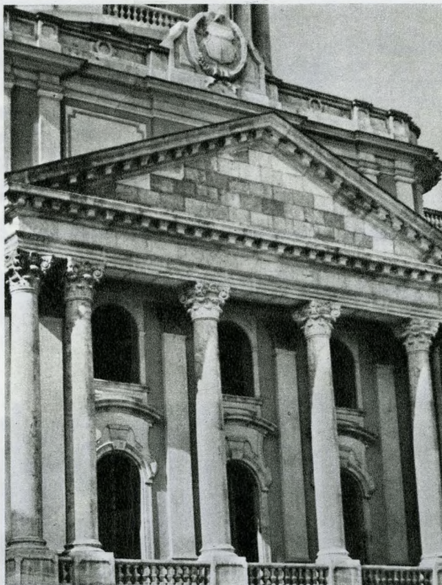
This palace will house the National Gallery. Its tympanum will be ornamented with bas-reliefs.
