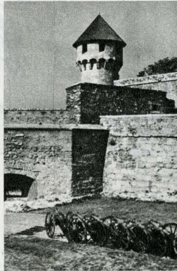
The southern bastion, built during the 15th century, had its defensive system worked out on three levels: the crenels of the battlement, the ramparts of the castle, and the flanking tower on the side.
