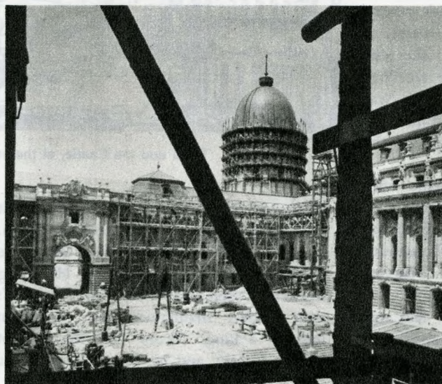
The court of honour, the so-called Lions' Court, will be reconstructed in its original Baroque style. Seventeen thousand pieces of carved stone were used for the restoration of this court with excellent acoustics, to be used for outdoor concerts, with a seating capacity of 3,000 people.
