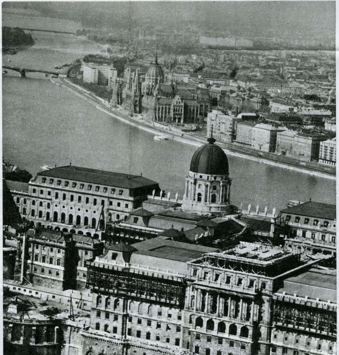
A view of the state of reconstruction. In the foreground the former royal chancery, which became after 1920 Horthy's residence and the governor's offices. It will house the National Library, covering 12 storeys with a shelf-place 400 kilometres long.
