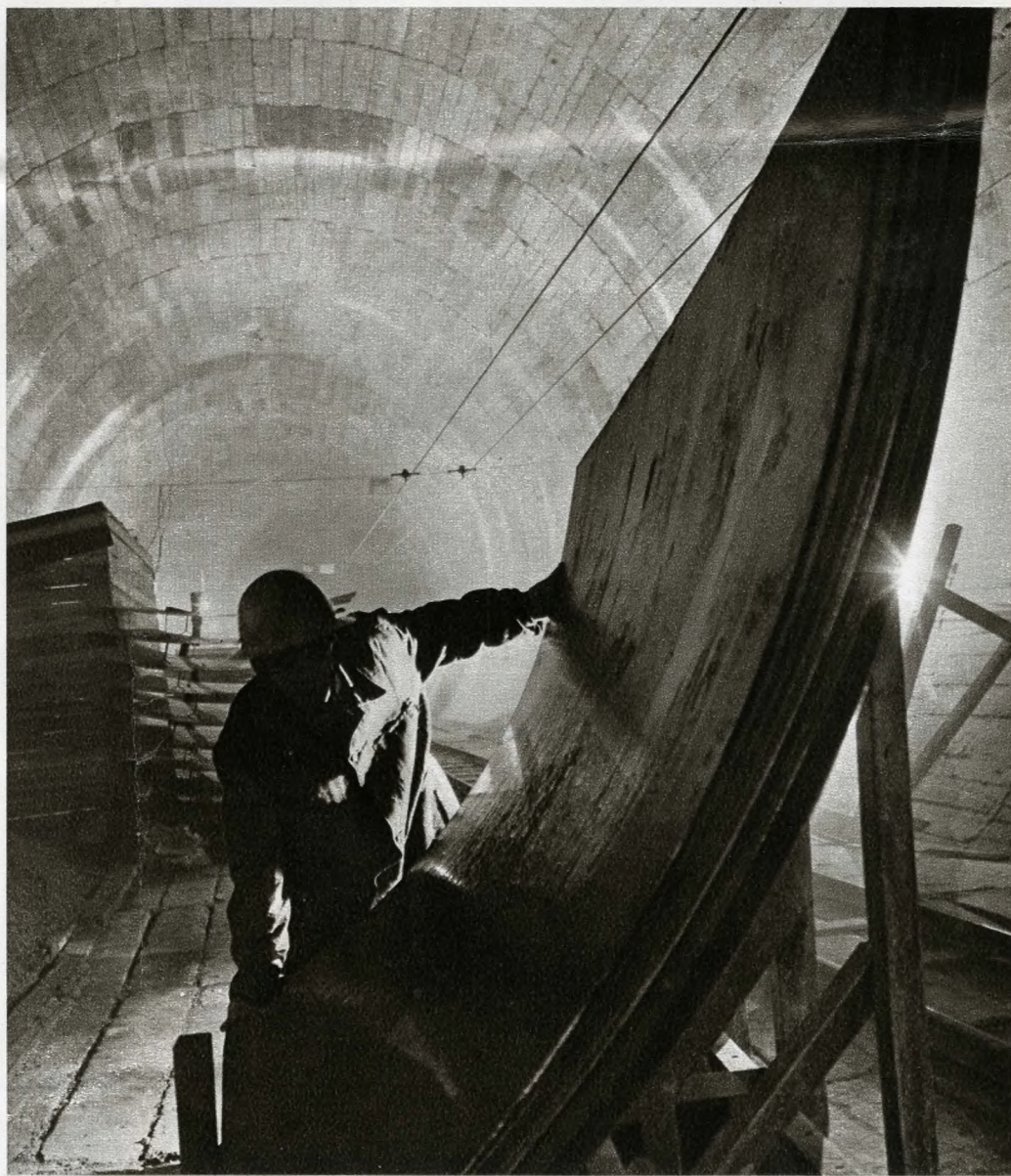
Preparing the iron sheets for insulation
