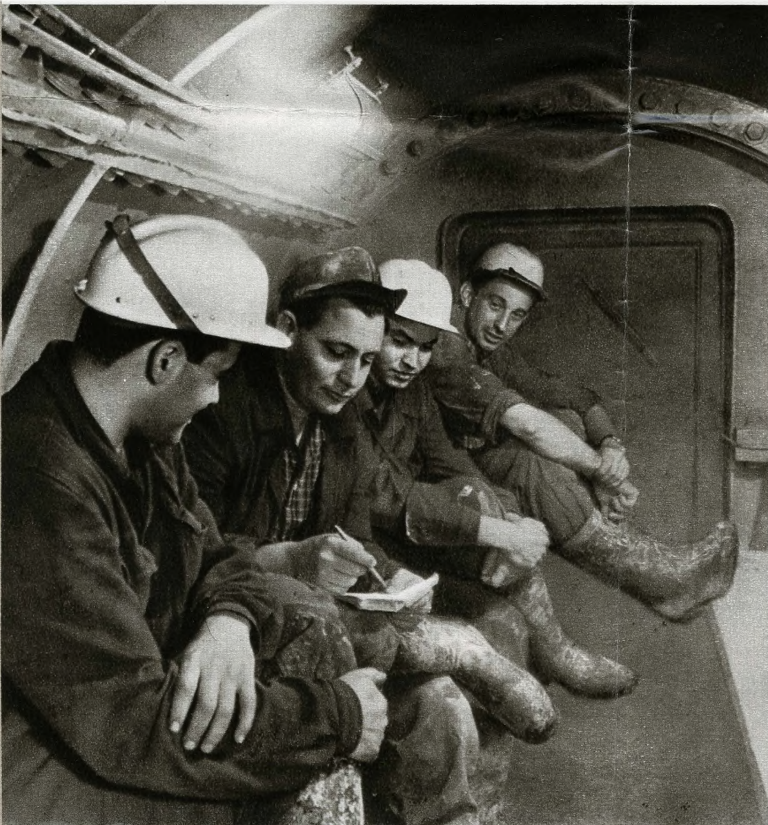
In the air-lock where they slowly level out the difference in atmospheric pressures
