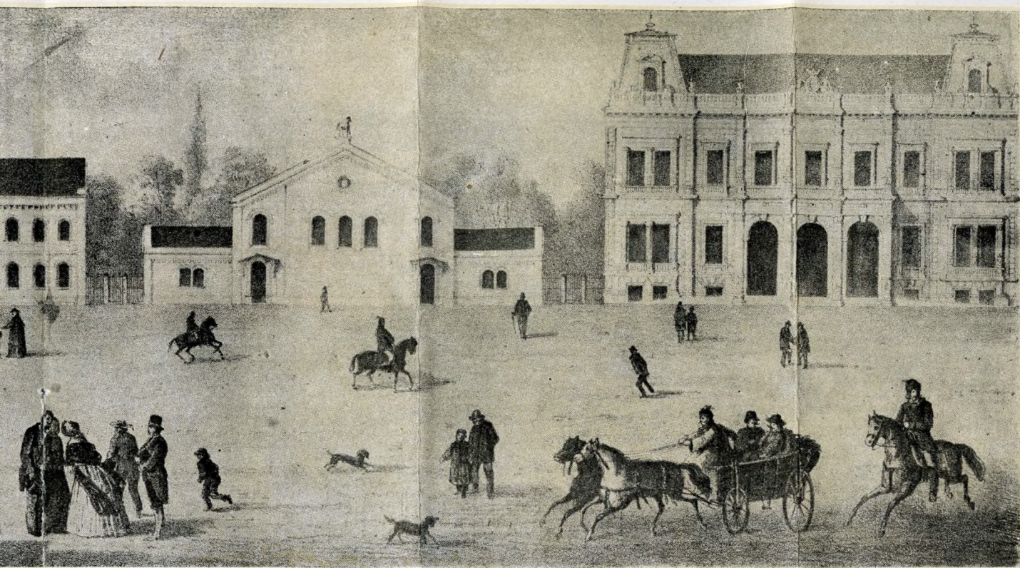
The buildings at the back of the National Museum (Designed and drawn by N. Ybl)
