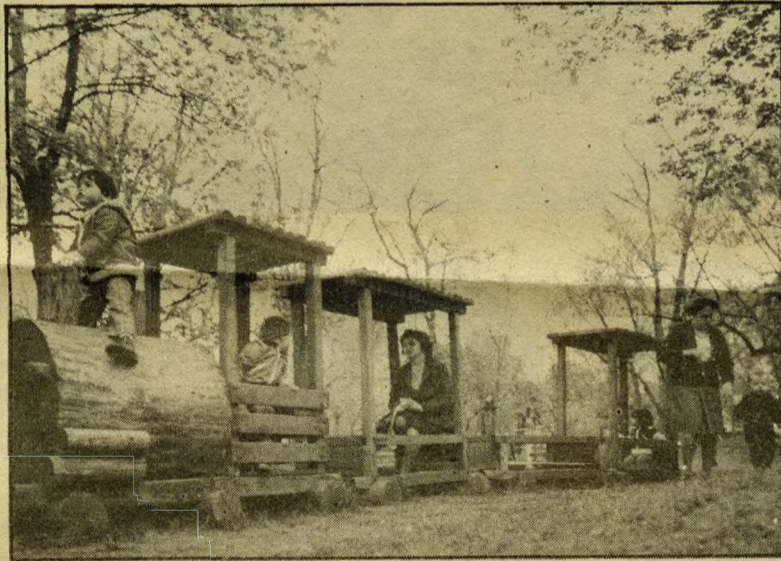
Log-and-boards structure imitating a train in the schoolchildren’s playground
